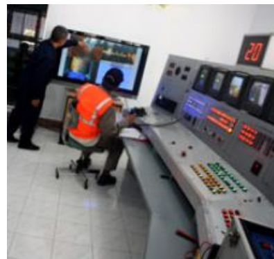
Gambar 4-2: Ground station di LAPAN Pameungpeuk
