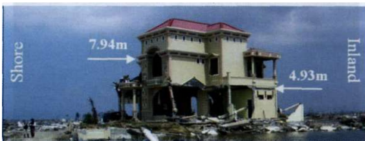
Fig. 9. Partially damaged family house located about 0.9 km inland in Banda Aceh. Left side is shore and right side inland. Numerals indicate inundation depths
