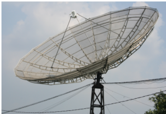
Gambar 3-1a: Antena penerima data HiRID
