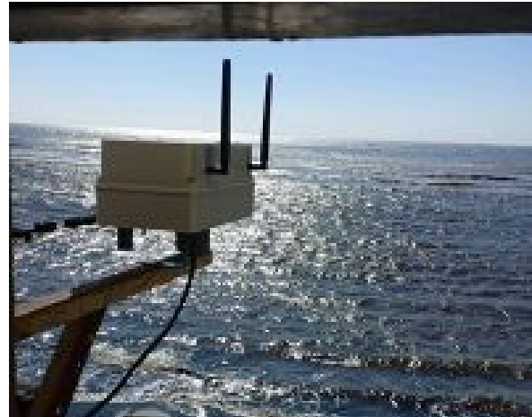
Figure 2. System installation at Banyuwangi.
