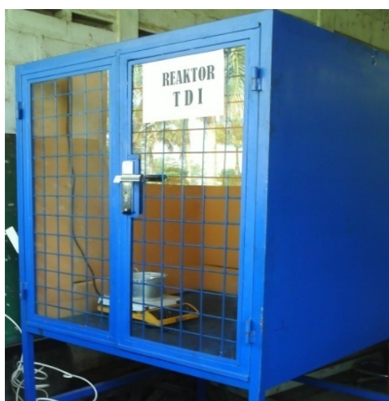
Gambar 4-4: Bunker proses TDA
